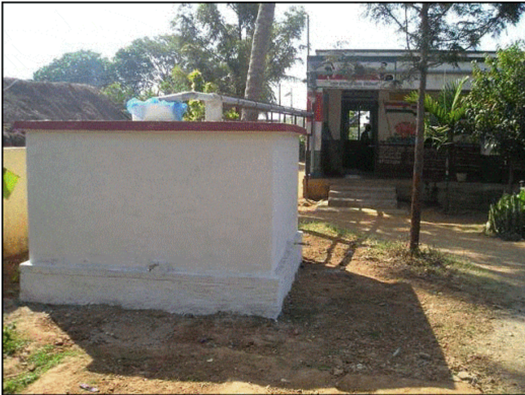
Fig ۷: A storage tank on a platform painted white
