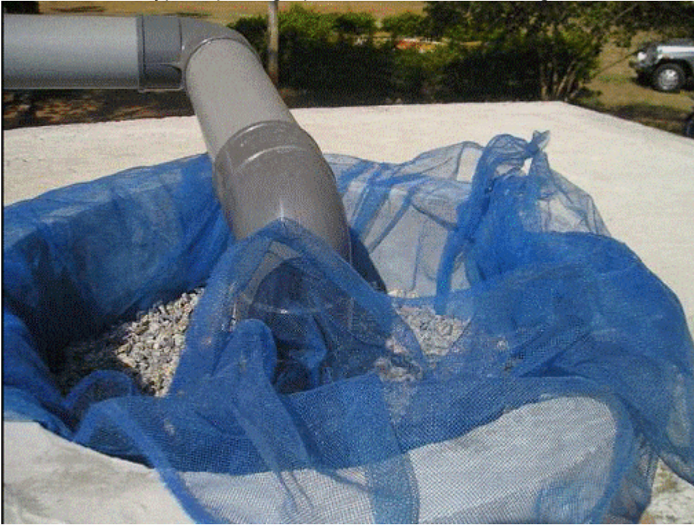
Fig ۲: Photograph of Typical Filter in Rainwater Harvesting
